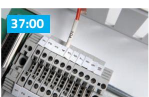
Wiring each terminal block one at a time.
