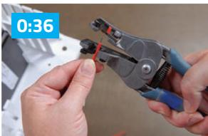
Continuing to measure and cut each control wire.
