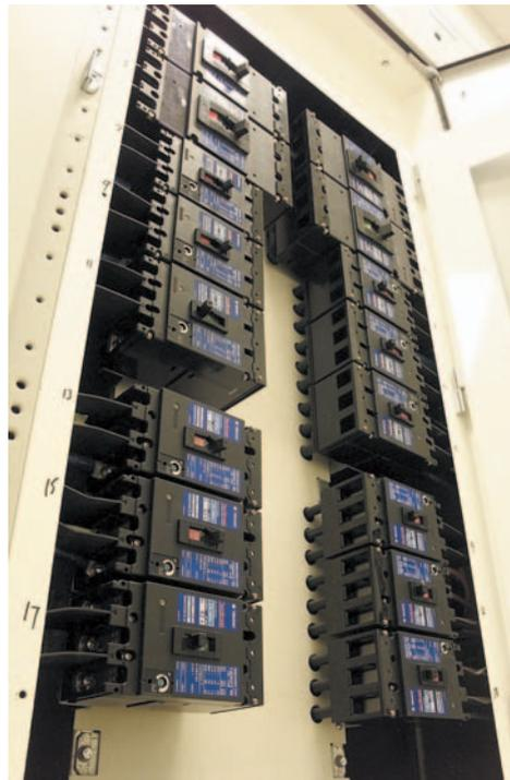
*Circuit Breaker assembly complying to Form 4bh. (When load-side terminal covers are fitted).*
