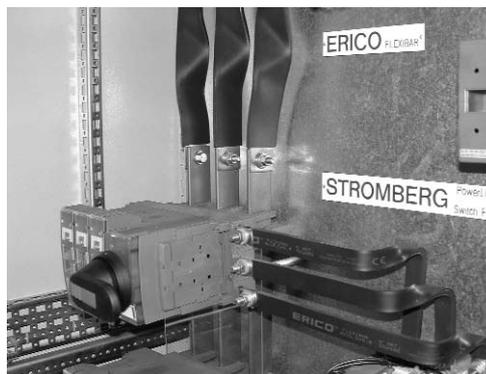
Flexible busbars can reduce assembly cost
