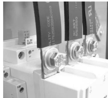
**Conductors connecting directly to switchgear should have a lower temperature rise**
