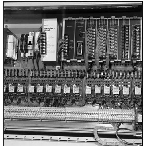
Failure can also start from poor contact pressure causing high resistance and hence high temperatures. Poor contact pressure may even result in the cable falling out of the connector.
