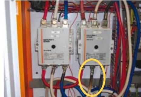
consequence, the tag did not sit square on the terminal thus creating a hot spot. The heat generated by this hot spot propagated through to the contact leading to premature failure.
