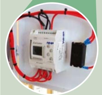
NHP used S&S contactors along with a Mitsubishi Alpha mini PLC to control the problematic water heating load to the research station in the North Canterbury bush
