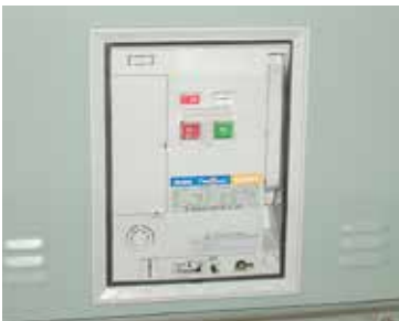
Completed retrofit of main circuit breaker
