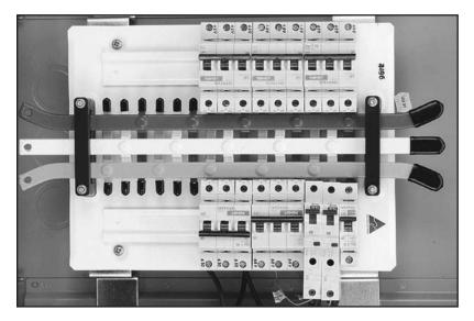
Single pole RCDs sit easily on chassis mount systems.
