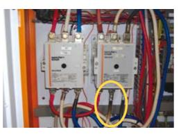
consequence, the tag did not sit square on the terminal thus creating a hot spot. The heat generated by this hot spot propogated through to the contact leading to premature failure.
