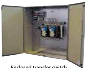
Enclosed transfer switch
