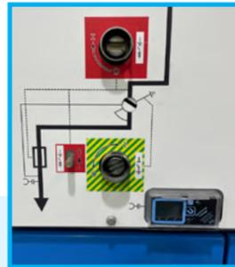
RV50 load break switch and earth switch which can both be padlocked in the open position
