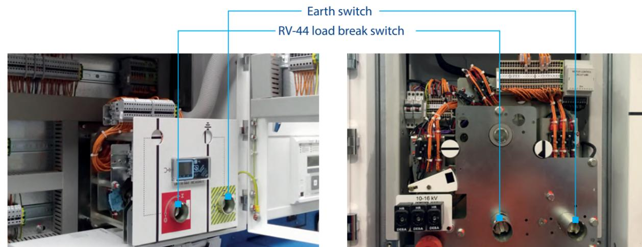
Mechanically interlocked earth switch and LBS with panel cover
