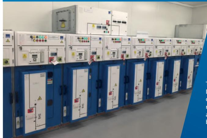
The example to the left shows a DF-D-EDN panel with a hinged door front mounted protection relay compartment. Above it is a horizontally mounted DF-LKB bus tie panel.
