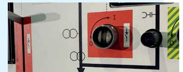
DF-2 panel with ISM VCB showing manual VCB opening lever
