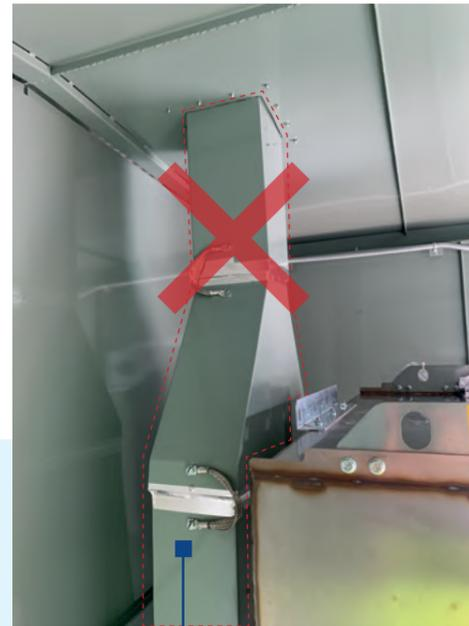
The need for gas chimneys is eliminated with DF2+, saving cost, space and simplifying installation
