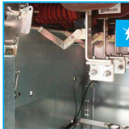
Internal Arc-Killer mechanism on the DF2+
