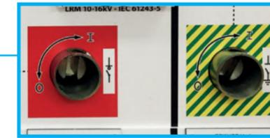
RV-44 load break switch (LBS) and earth switch, which can both be padlocked in the open or closed position
