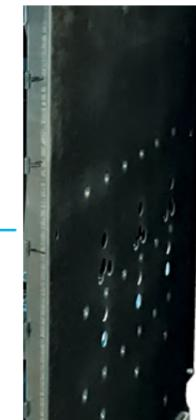
2mm thick steel walls ensuring internal arc fault containment within the compartment where it has originated
