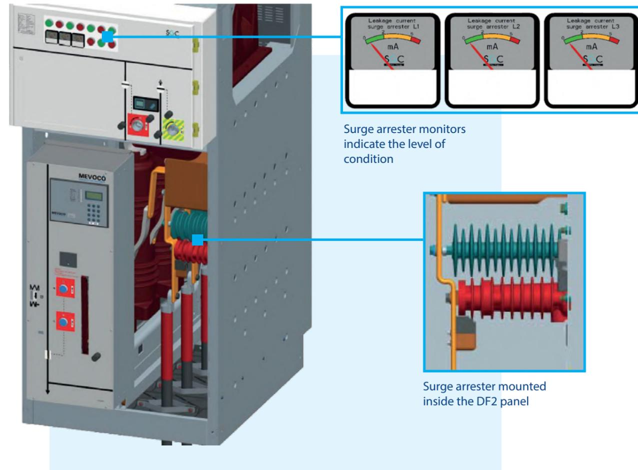
Surge arrester monitors indicate the level of condition
