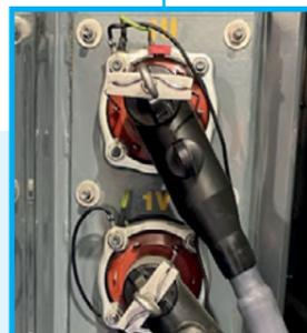
HV plug-in bushing for safety
