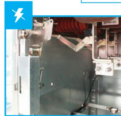
Internal Arc-Killer mechanism on the DT-6+
