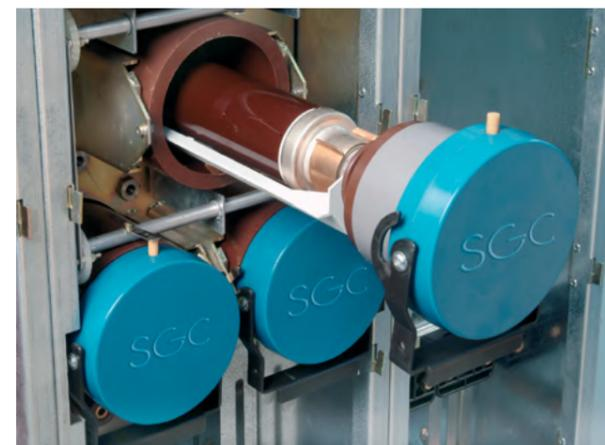
MV panel with ISM VCB showing manual VCB opening lever
