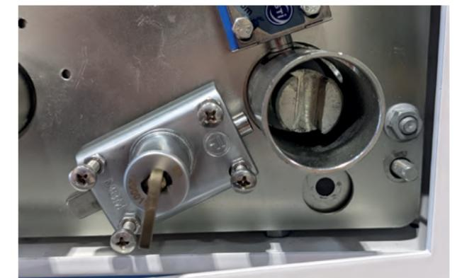
Ronis key interlock fitted to LBS/ESW panel
