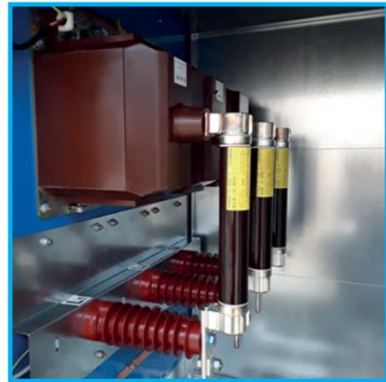
Fuses can also be used for protection instead of the VCB
