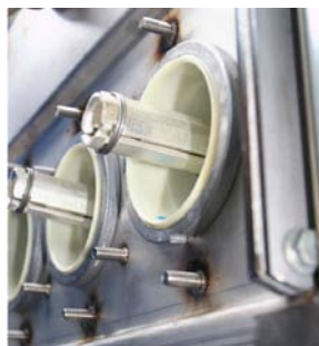
Figure 10: Busbar extension
