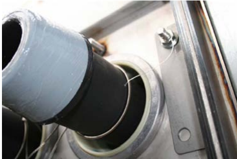
Figure 13: Ground connection
