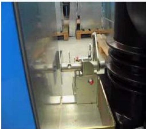
Photo 10: drilling in main axis of arc-killer
