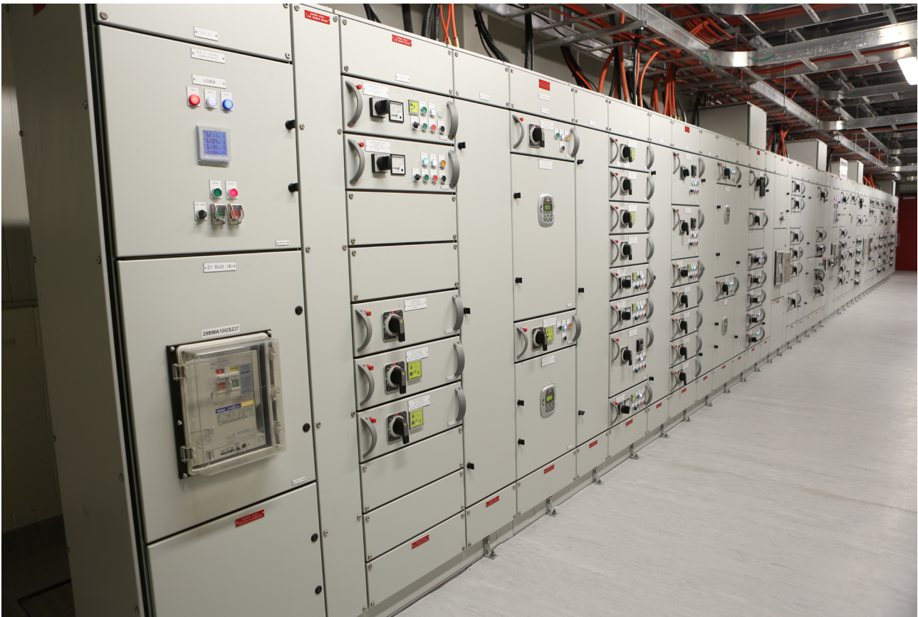
Above: Typical switchboard with power distribution and motor control elements
