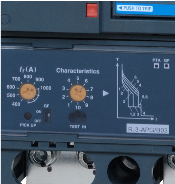
Figure 3.4.9 Top: Dial setting 10 disables the thermal and short time instantaneous portion of the curve
