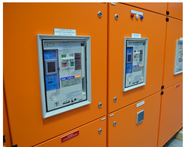
Figure 3.2.1 ACBs fitted in a Main Switchboard
