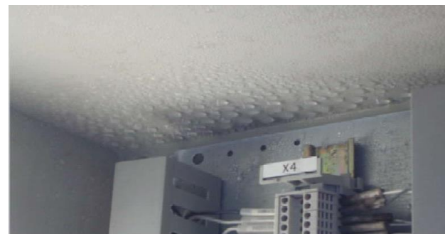
Internal top panel of an IP66 enclosure
