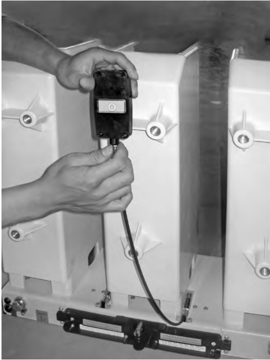
Figure 62 Adjust the indicator for both closed and opened states of the switching module.
